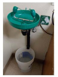
Photo 2: Several sites had eyewash stations that did not drain to plumbed sewer lines. These stations are not amenable to flushing and their use would likely result in exposing the worker's eyes to high bacterial loads. It is also likely that employees would rinse for less than the necessary time out of fear of overflowing the container.
