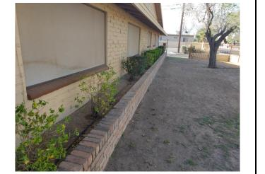
Photo 5: Planters, etc. that are directly against the building can retain moisture, degrade the structure, promote termite establishment, and cause water infiltration if not properly drained.
