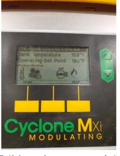
Photo 7: The ideal water tank temperature to prevent Legionella is above  $140^{\circ}$ F.
