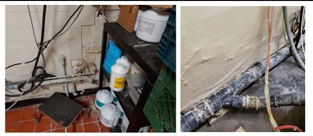
Photo 17: Water damaged wall systems are a common site in laundry and kitchen areas. Walls and floors in these areas should be as waterproof and chemical resistant as possible. Placing water resistant surfacing over water sensitive materials often causes more harm than good, as water "finds a way", wicks up the susceptible material, and is trapped for an extensive time, allowing for degradation and mold development.
