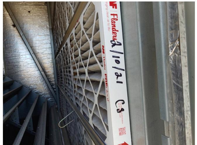
Photo 6: Labeling filters with the date of installation is especially helpful to those encountering filters in the field
