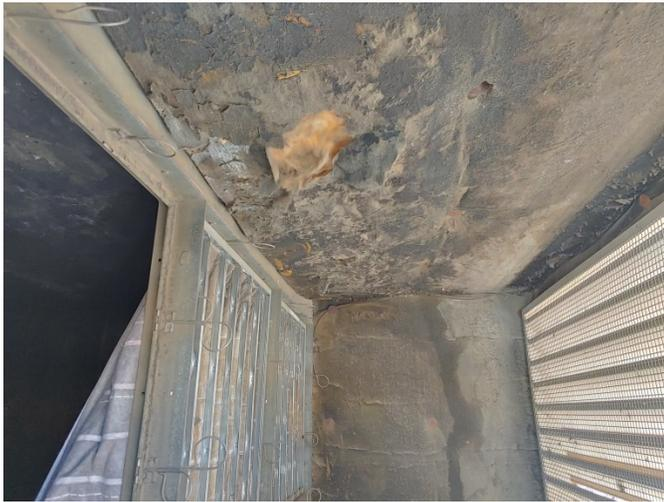
Photo 18: HVAC units and plenums should be regularly inspected and repaired when needed. Degraded HVAC duct lining and plenums will entrain and distribute potentially hazardous materials.
