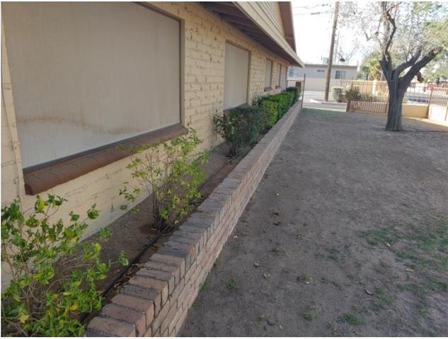
Photo 5: Planters, etc. that are directly against the building can retain moisture, degrade the structure, promote termite establishment, and cause water infiltration if not properly drained.
