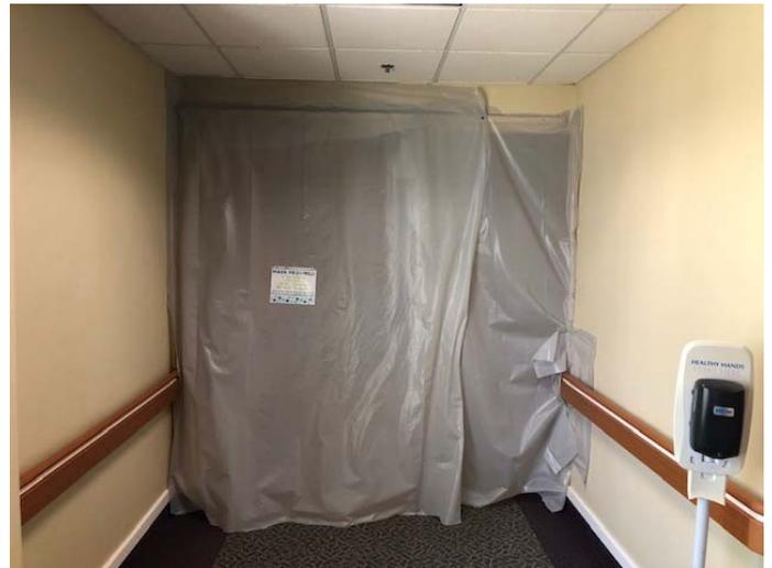
Photo 12: Isolation / quarantine areas should be under negative pressure to prevent the release of airborne pathogens into common areas.
