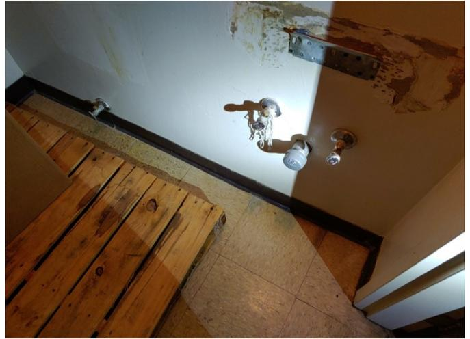
Photo 10: Abandoned plumbed areas require regular flushing or termination at the main water line to prevent water stagnation and Legionella development.
