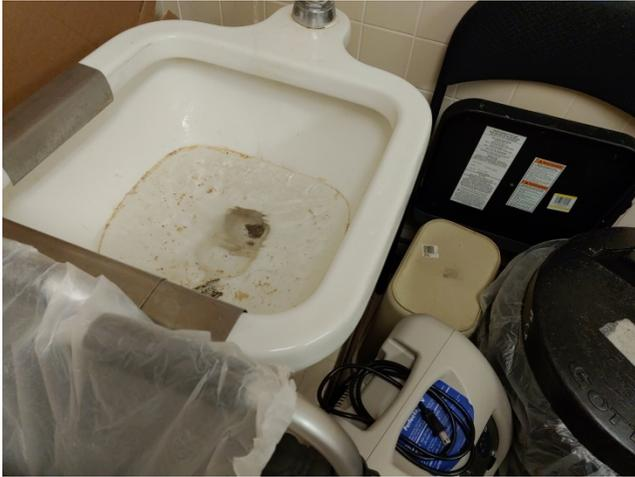
Photo 1: It was common to find utility sinks called “hoppers” which failed to drain or were inoperable. This becomes a sanitary issue and a legionella issue because the fixture cannot be effectively flushed.
