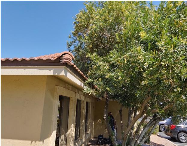
Photo 3: Vegetation that touches the roof or extends beyond it becomes a route for rodent entry and can cause drainage issues on flat roofs due to leaf litter accumulation.
