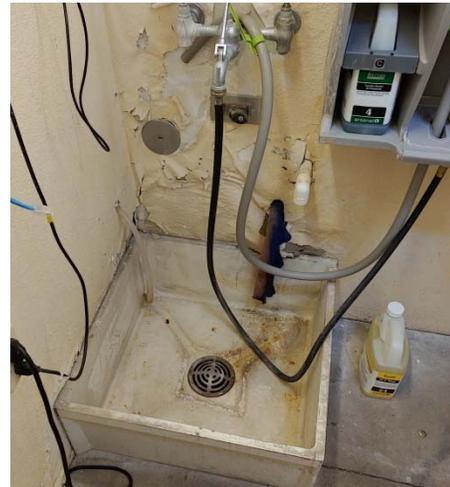
Photo 16: Water use areas should incorporate splash guard and waterproof construction.
