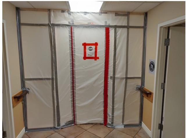
Photo 2: This isolation wing was properly under negative pressure compared to the common hallway.
