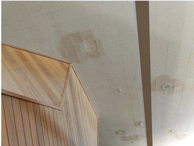
Photo 11: Replacing stained ceiling tiles will help diagnose roof or condensation leaks, removes potential mold sources, and presents an aesthetic of cleanliness.
