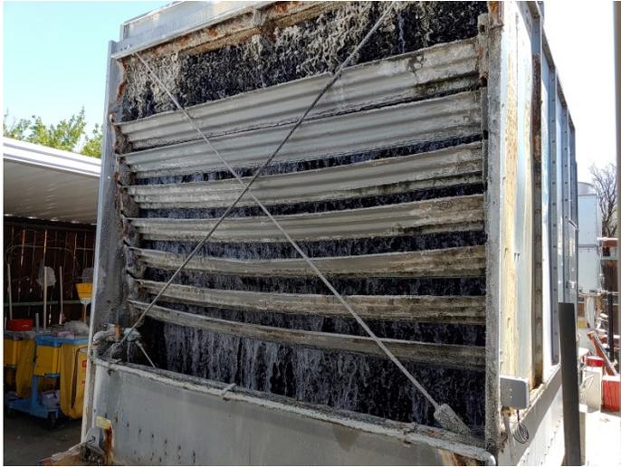
Photo 9: Cooling towers must be maintained to be in the best condition possible, to prevent the release of bioaerosols which may contain Legionella.
