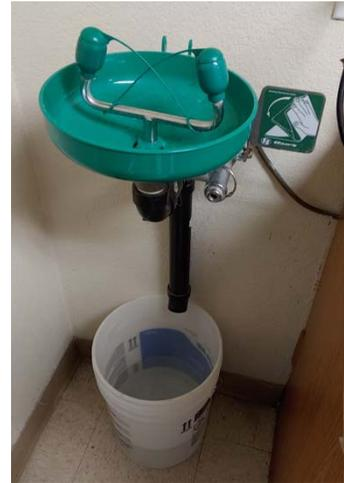
Photo 2: Several sites had eyewash stations that did not drain to plumbed sewer lines. These stations are not amenable to flushing and their use would likely result in exposing the worker’s eyes to high bacterial loads. It is also likely that employees would rinse for less than the necessary time out of fear of overflowing the container.
