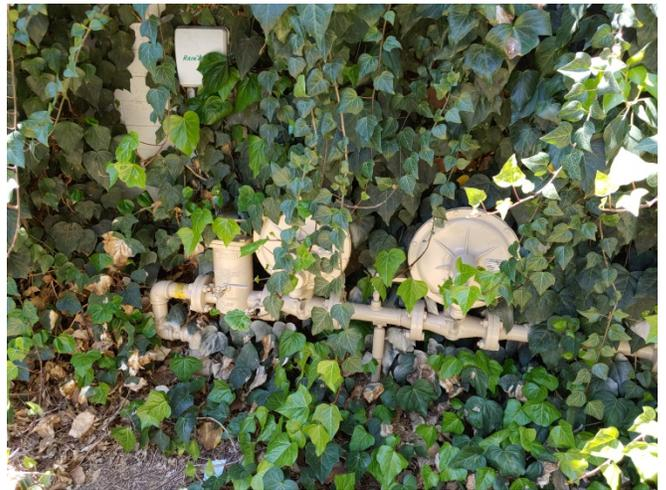
Photo 4: Vegetation against the building becomes pest habitat, traps moisture, and inhibits visual inspection of the building exterior.
