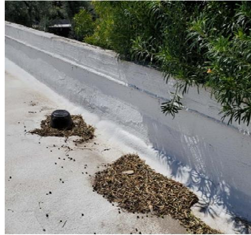
Photo 14: Flat roofs require frequent inspections and clearing to prevent drain blockage and flow damming. Trees should be trimmed to reduce leaf litter accumulation and eliminate pest pathways.
