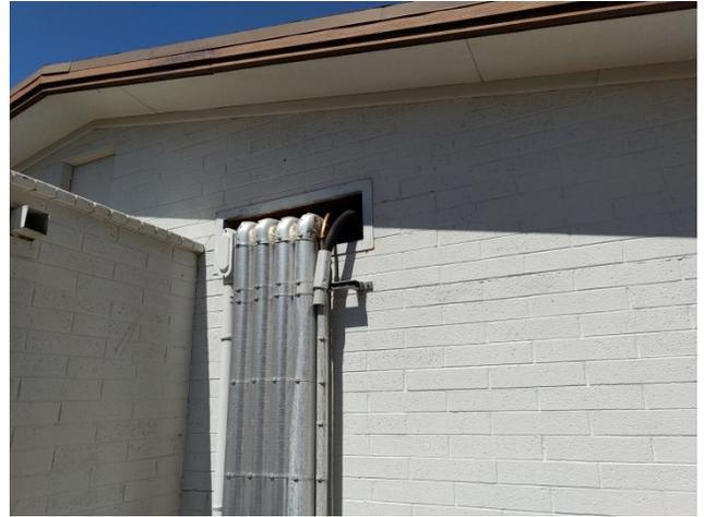
Photo 6: All exterior penetrations should be sealed or include pest barriers.
